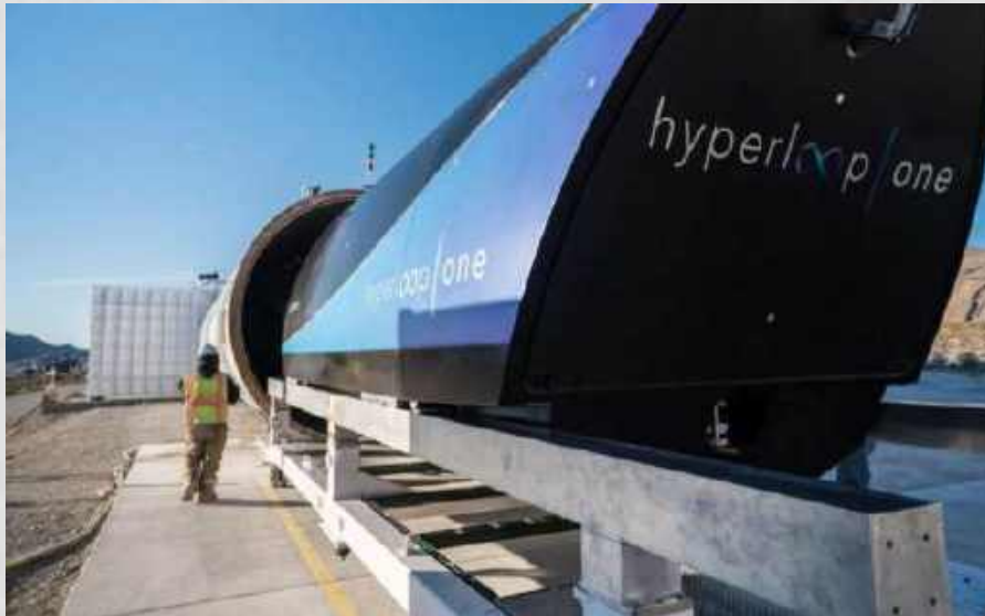
Fig. Hyperloop construction.
