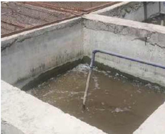
Step 3: Secondary treatment (Aeration / Activated Sludge)
